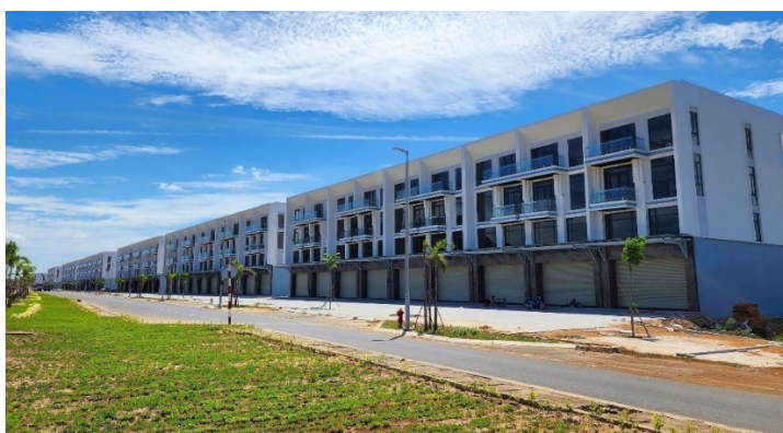
Figure 10: Sonadezi Huu Phuoc project
