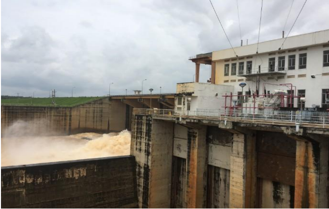
Figure 15: Srok Phu Mieng hydropower plant
