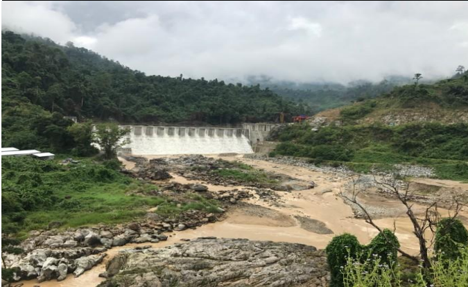
Figure 16: Dak Mi 3 hydropower plant
