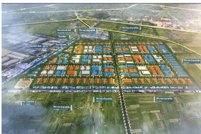
Figure 10: Tan Phuoc 1 IP, take advantage on rising infrastructure development
